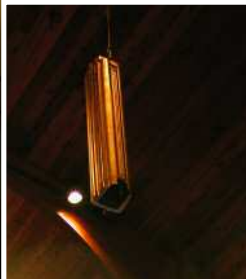
To the left, one of the underbalcony loudspeakers serving shadowed regions, and above, a rear view of one of the DSA250 mains.
