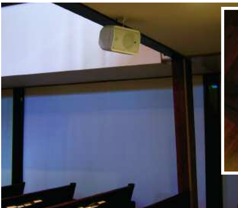
To the left, one of the underbalcony loudspeakers serving shadowed regions, and above, a rear view of one of the DSA250 mains.
