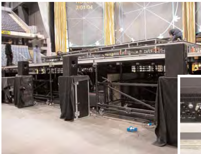
Wide-coverage loudspeakers on road cases for front fill, and (right) clean I/O from the house console.
