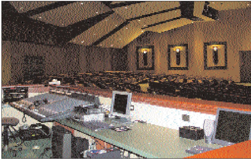
The system control position, located at the rear/center of the audience area, anchored by a Yamaha M2500 console.
