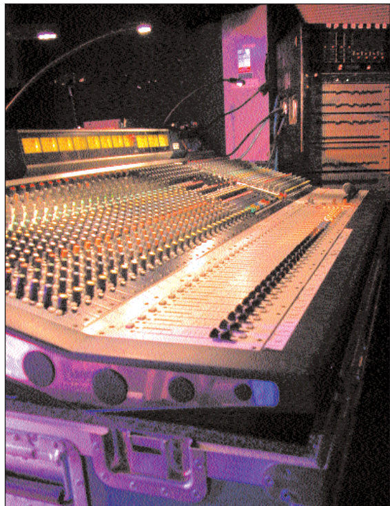
One of the MH4 consoles, this one on stage for monitoring. Plenty of channels of Klark-Teknik third-octaves available as well.
