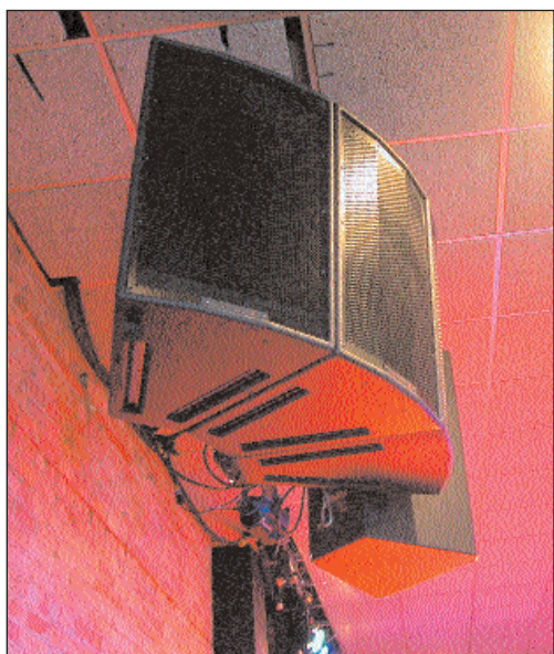
One of the house arrays, with stage fill speaker flown behind.
