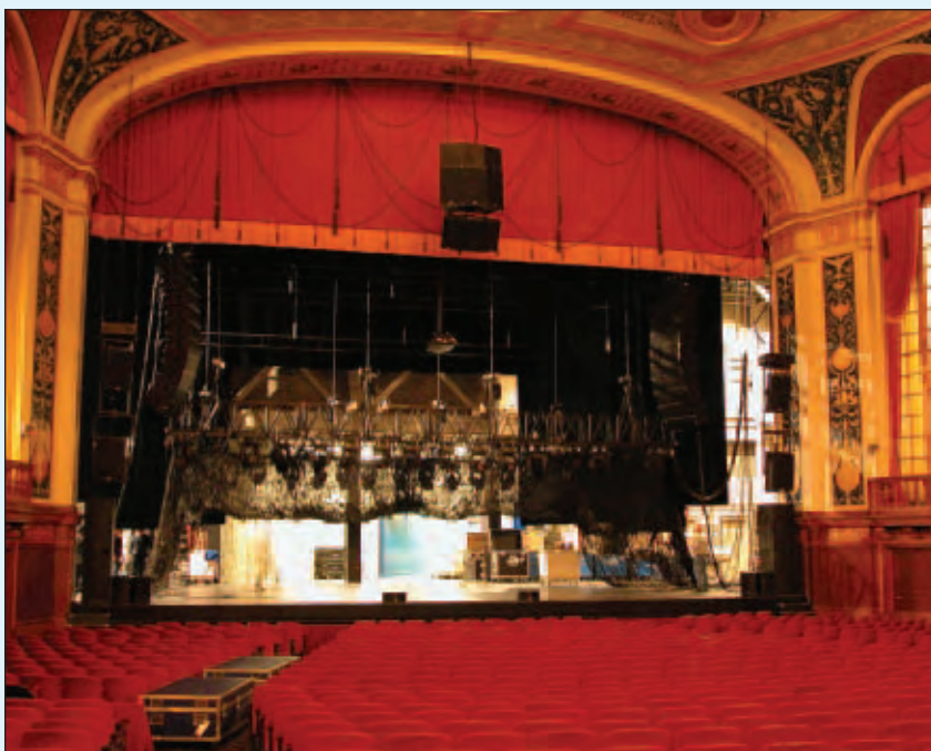
As the installed left-center-right house system looks on helplessly, the full-scale concert system for Izzard goes into place.
